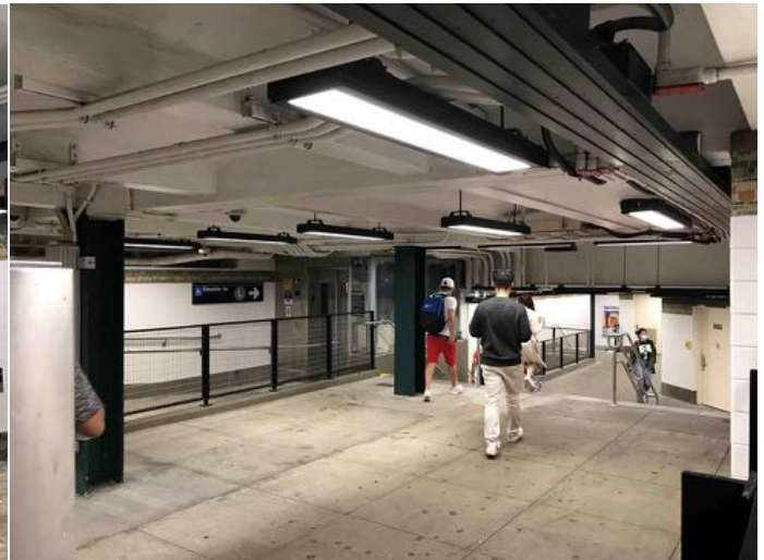
View looking east at the expanded Bedford Avenue mezzanine, with the mezzanine to platform elevator in the center-left, and a short set of steps down to the two platform stairs, with one immediately visible to the right and the second one just visible beyond. This photo was taken from just outside the paid fare zone, as I was leaning on the railing. This entire expanded mezzanine was excavated and constructed in a cut and cover operation from the street. Note the ramp leading down to the elevator that was required to obtain the necessary headroom for the elevator's installation.
