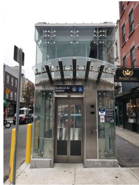
A head-on view looking north at the new elevator on the east sidewalk of Bedford Avenue at the corner of North 7th Street.
