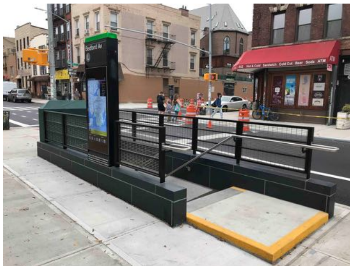
The new stair on the northeast corner of Driggs Avenue and North 7th Street, oriented north along the east sidewalk of Driggs Avenue. Note the vertical digital information display, the stair enclosure, and railing are all in a style similar to what has been installed at stations rehabilitated under the Enhanced Station Initiative.
