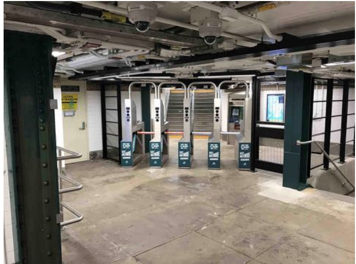
Driggs Avenue mezzanine, view looking northeast at the fare array. Beyond that is the new diagonal street stair, rising to an intermediate landing from which are two stairs to each side of the northeast corner of Driggs Avenue and North 7th Street. An identical fare array and street stair arrangement is out of view to the right. The top of the new P6 platform stair is visible at right.
