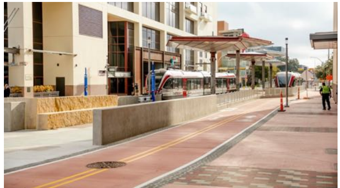
The new MetroRail Downtown station. The station also features parasol structures mounted on columns, offering a striking visual welcome to downtown and overhead protection for customers as they wait for, enter or exit the train cars.
