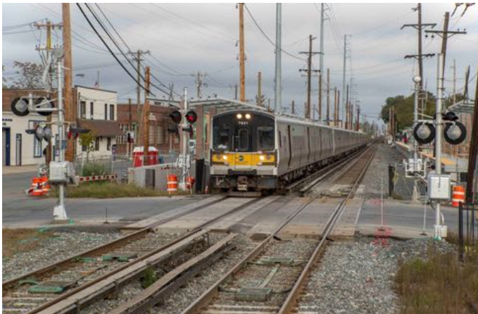
Another view taken on October 23, this one looking east from the temporary eastbound platform at the New Hyde Park station. Huntington-to-Penn Station Train #1705, with M-7 7621 (Bombardier Transportation, 3/2006) leading, passes over the South 12th Street grade crossing. On the far side of the crossing are the new, still-under-construction, permanent platforms. Note the space provided on the right for the future third track.
