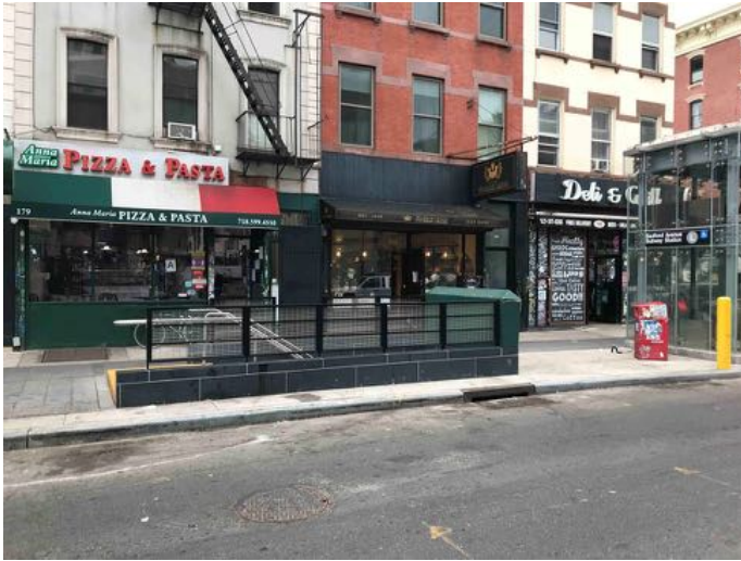
View of the new street stair and elevator on the east sidewalk of Bedford Avenue just north of the corner of North 7th Street.
