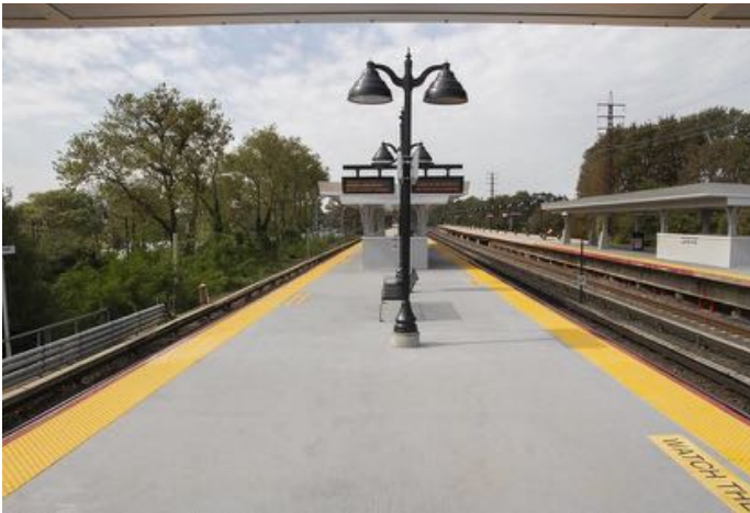
Upgraded Platform B, serving the Long Beach Branch, at Lynbrook on October 7.
