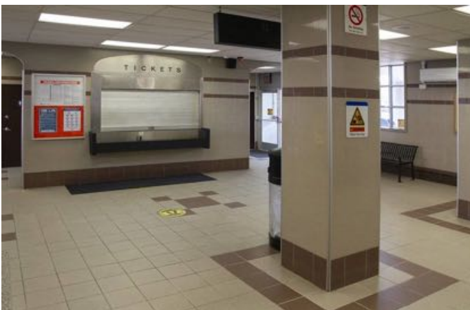
Rebuilt ticket office and waiting room.
