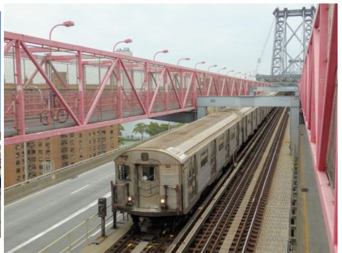
Train of R-32s southbound on Williamsburg Bridge.
