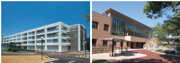
Rehabilitation centers in Nakaizu (left) and Beppu (right)
