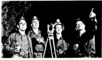
On the 50 level while on an inspection tour, Mine Engineer Don McLeod and Little Stobie Mine Superintendent Sam Pataran are seen with Survey Assistant Gerry MacIsaac and Layout Engineer Charile Pitts. The survey instrument was being used to install lines for ring drilling.
