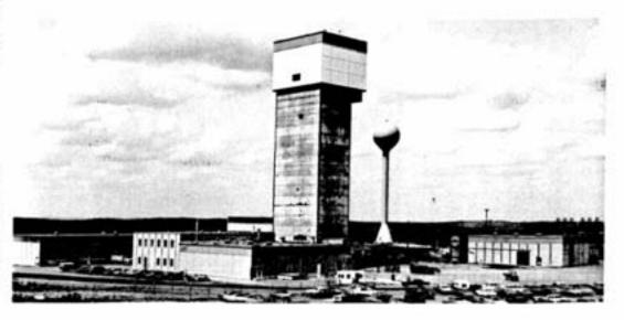
Efficiently grouped around the base of the concrete headframe, Little Stoble's surface plant buildings contain administrative and engineering offices, changehouse with facilities for 452 men, coltarhouse and warm room. A warehouse and maintenance shop are on the left, a compressor house on the right. Its shape identifying the mine from the many others in the district, the streamlined water tower holds 100,000 gallons.
