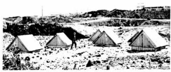
Each of these huts houses the upper ends of six stalnless steel wires. The lower ends of the wires are anchored in the hangingwall close to the Little Stoble crebody on the 100-, 150-, and 200-toot levels. A ground control system, they monitor rock movement during the preliminary stages of sub-level caving. Using extensometers to measure changing strains in the wires, engineers are able to plan precisely controlled caving of the hangingwall rock.
