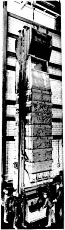
In the collarhouse at Frood-Stoble No. 9 shaft, this is one of the 20-ton bottom dump skips, largest in the Ontario Division, In which Little Stoble Mine ore is hoisted to the Frood-Stoble Mill storage bins. Operated by a 4.200-h.p. 4-rope friction hoist, the skip travels at 3,000 feet per minute. Dwarfed beside the huge conveyance are Riggers Frank Kuznik, Moses Roy, Tony Pinard and Gerry Vincent.
