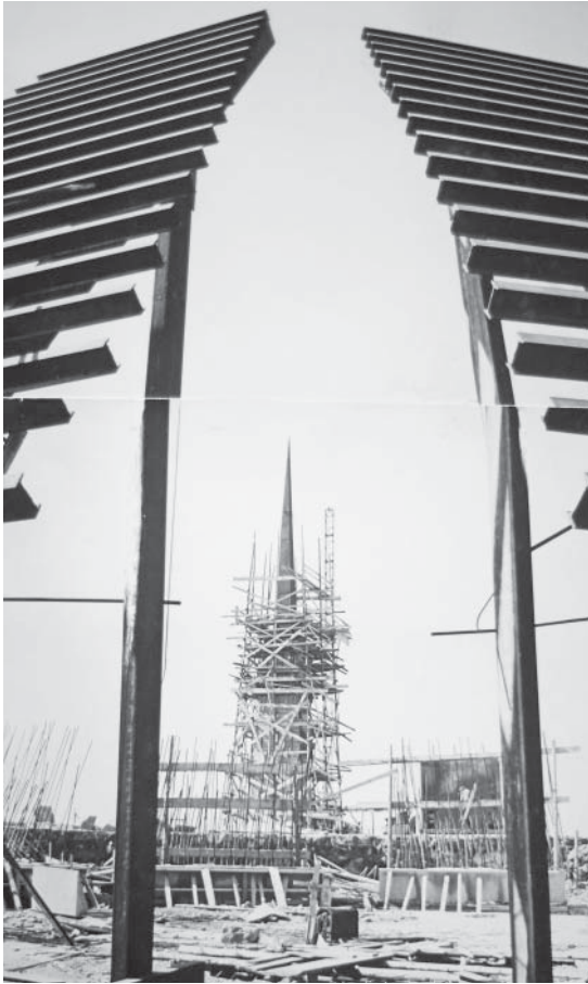
Construction work at the Genocide memorial complex, 1966
