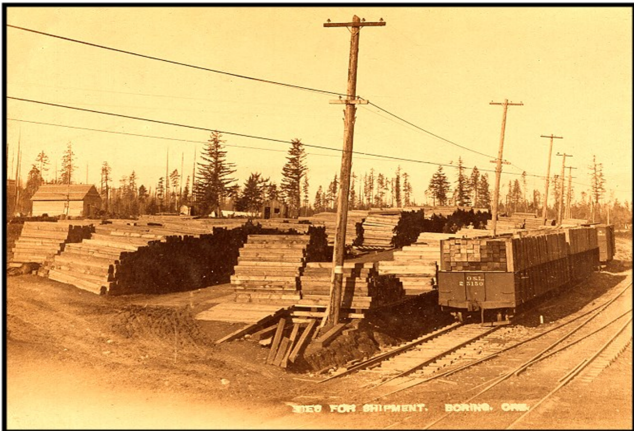
Early post card view of ties cut and ready for loading at the lumber mill in Boring. Post card courtesy of Steve Kenney.
