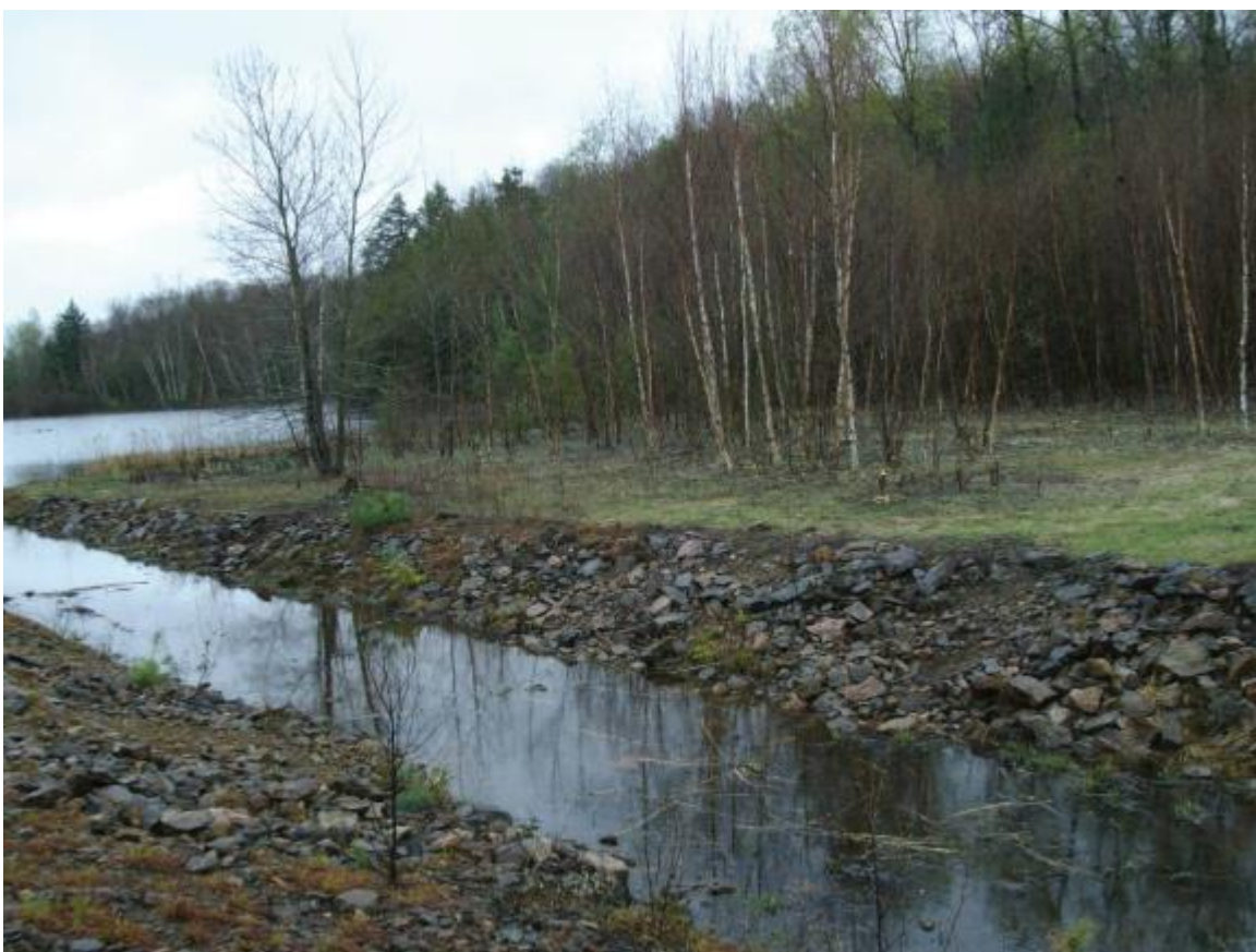
Figure 8.9: South tailings basin spillway at Bicroft tailings storage facility
