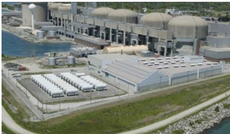
Figure 5.1: Pickering Waste Management Facility with retube components storage area (left) and spent fuel dry storage area (right)
