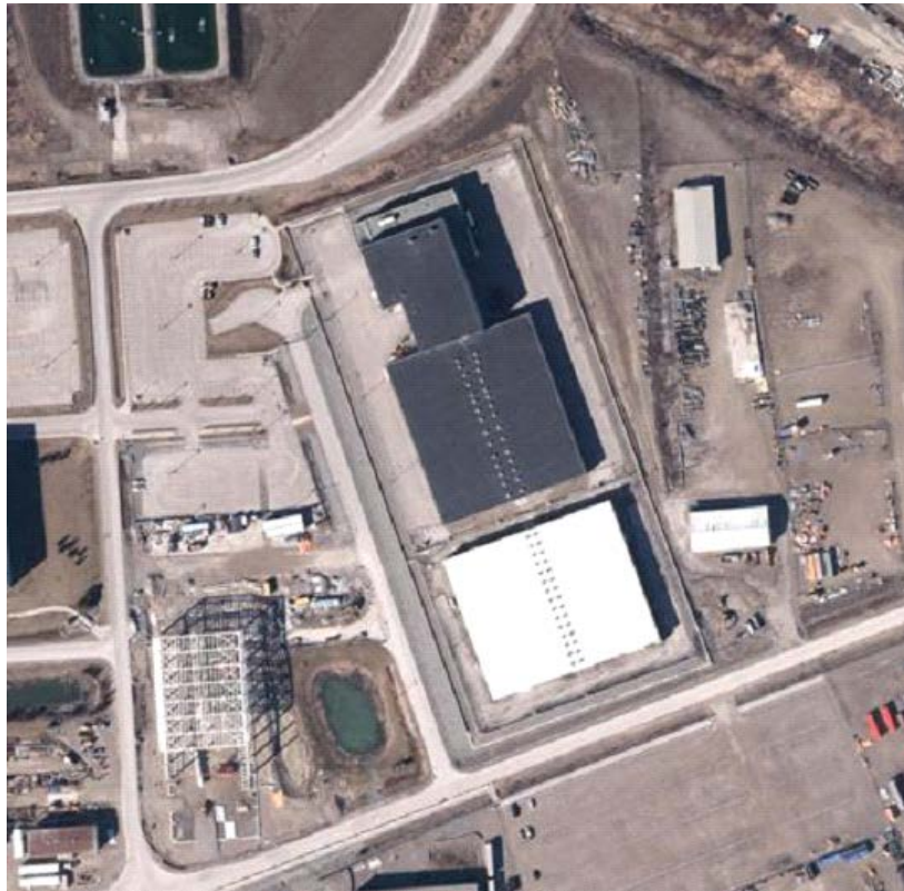
Figure 4.6: Aerial photo of the Darlington Waste Management Facility
