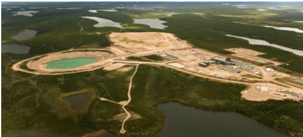
Figure 6.3(a): McClean Lake operation with John Everett Bates tailings management facility located to the left of the mill
