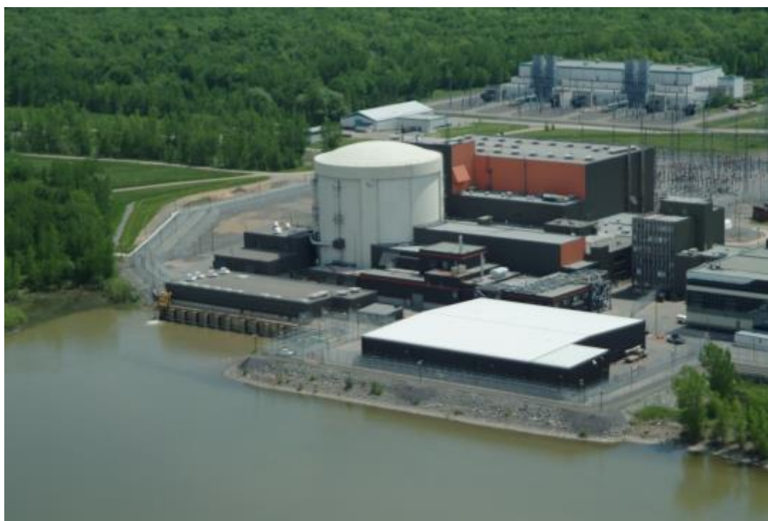
Figure 4.7: Gently-2 Nuclear Generating Station
