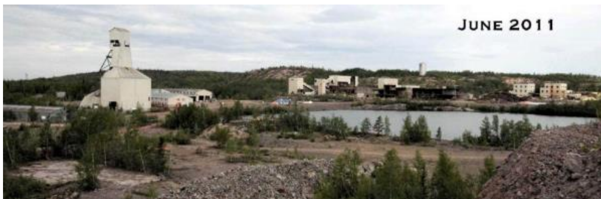
Figure 8.3: Before completion of the CNSC order
