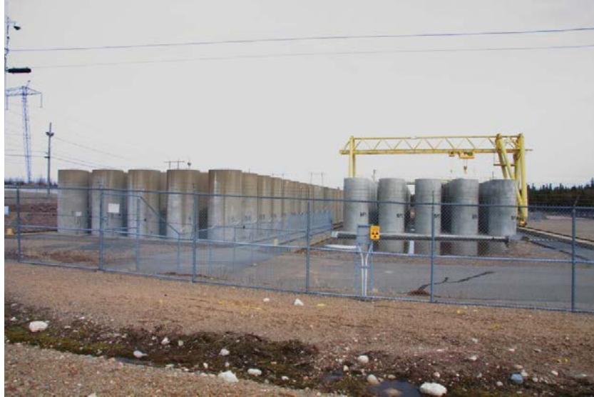
Figure 4.9: Point Lepreau spent fuel dry storage facility area
