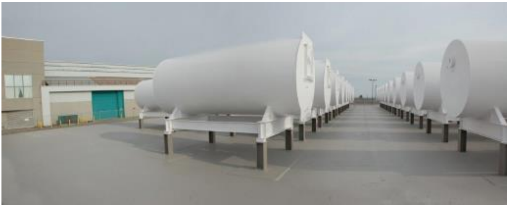
Figure H.1: Dry storage modules containing Pickering A (Units 1 to 4) retube waste at the Ontario Power Generation's Pickering Waste Management Facility (PWMF)
