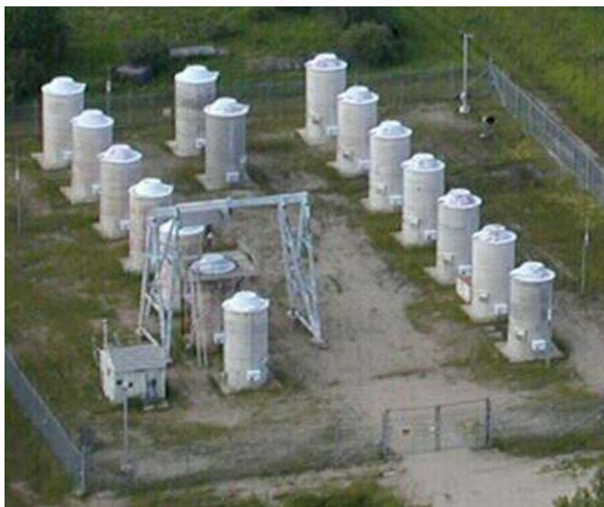
Figure 4.11: Whiteshell Laboratories Concrete Canister Storage Facility
