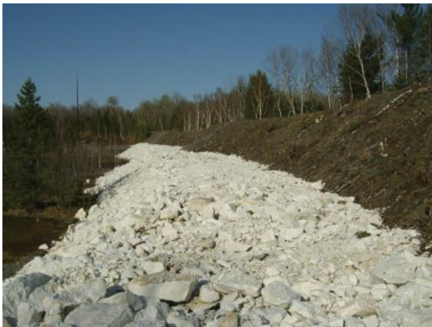
Figure 8.8: Main tailings dam, Dyno mine site
