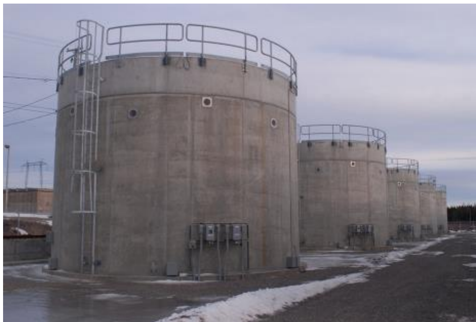
Figure 5.5: Point Lepreau retube waste canisters
