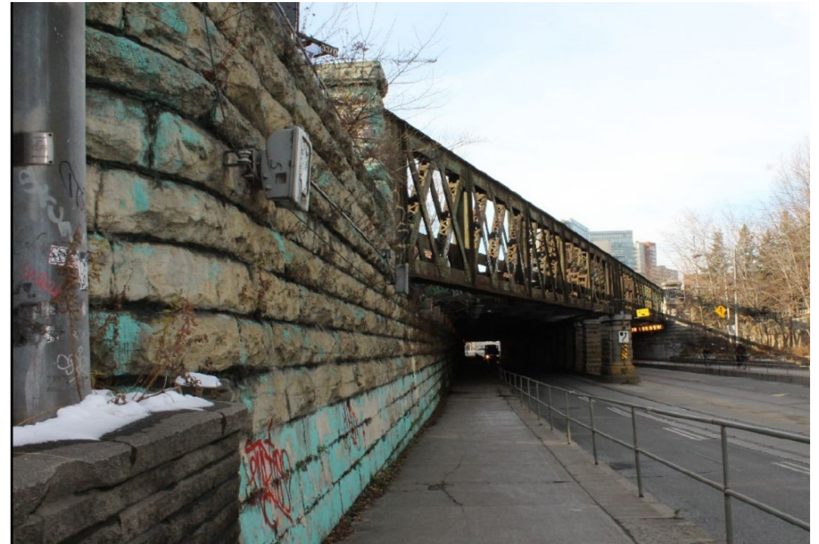
King St. W. Subway, looking west along King St. W
