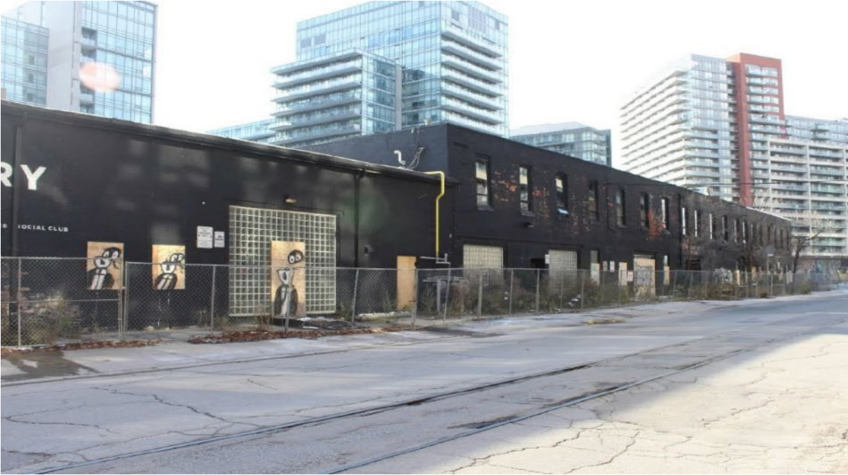
North façade of 99 Sudbury St.
