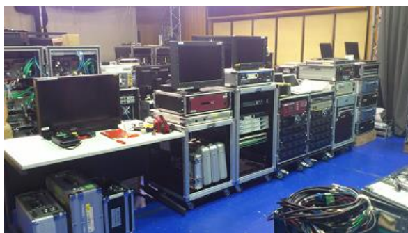
Line and transmission equipment
