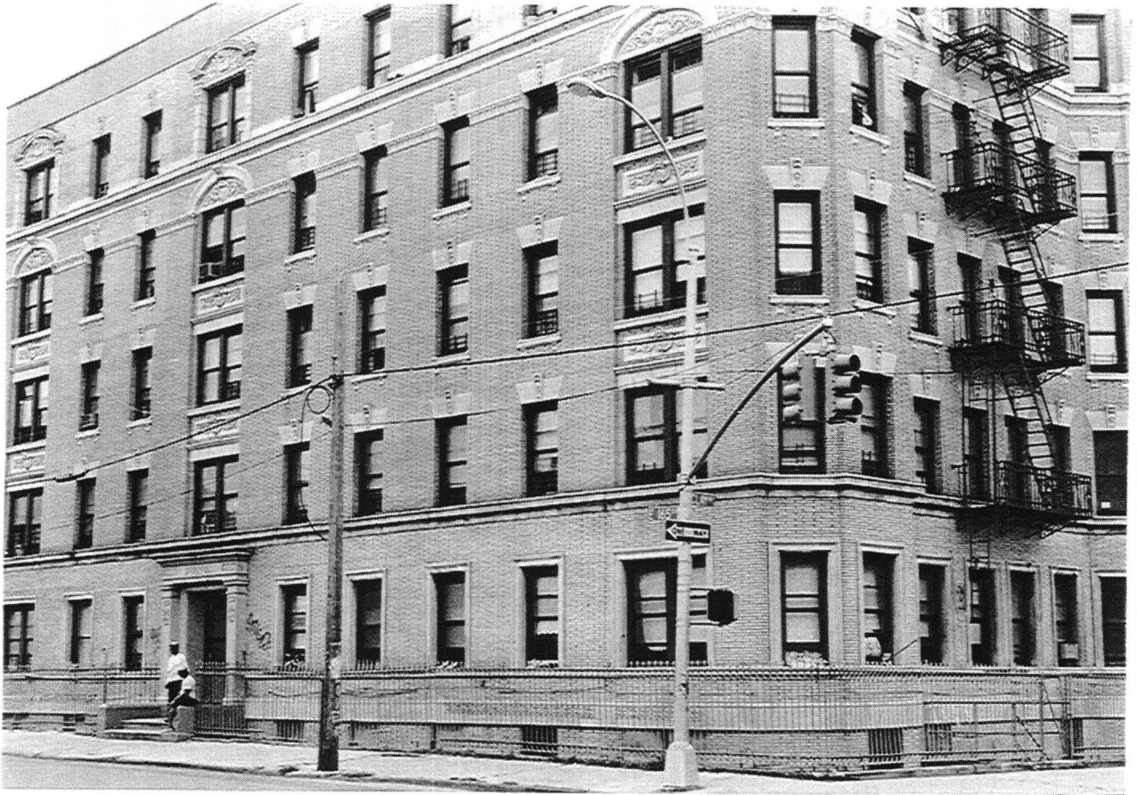
371 East 165th Street, aka 1039 Clay Avenue
