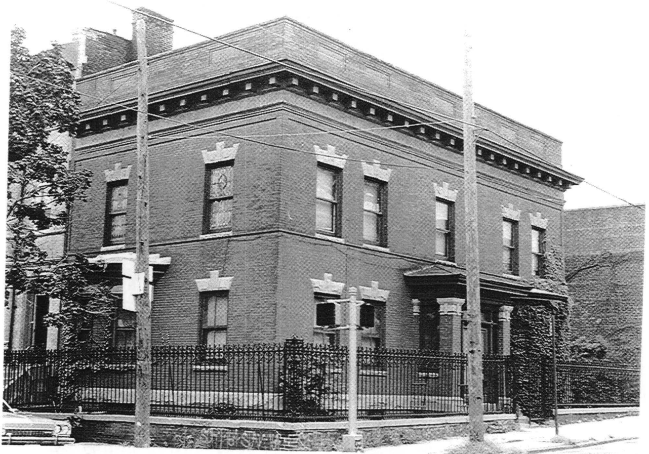
381 East 165th Street, aka 1038 Clay Avenue
