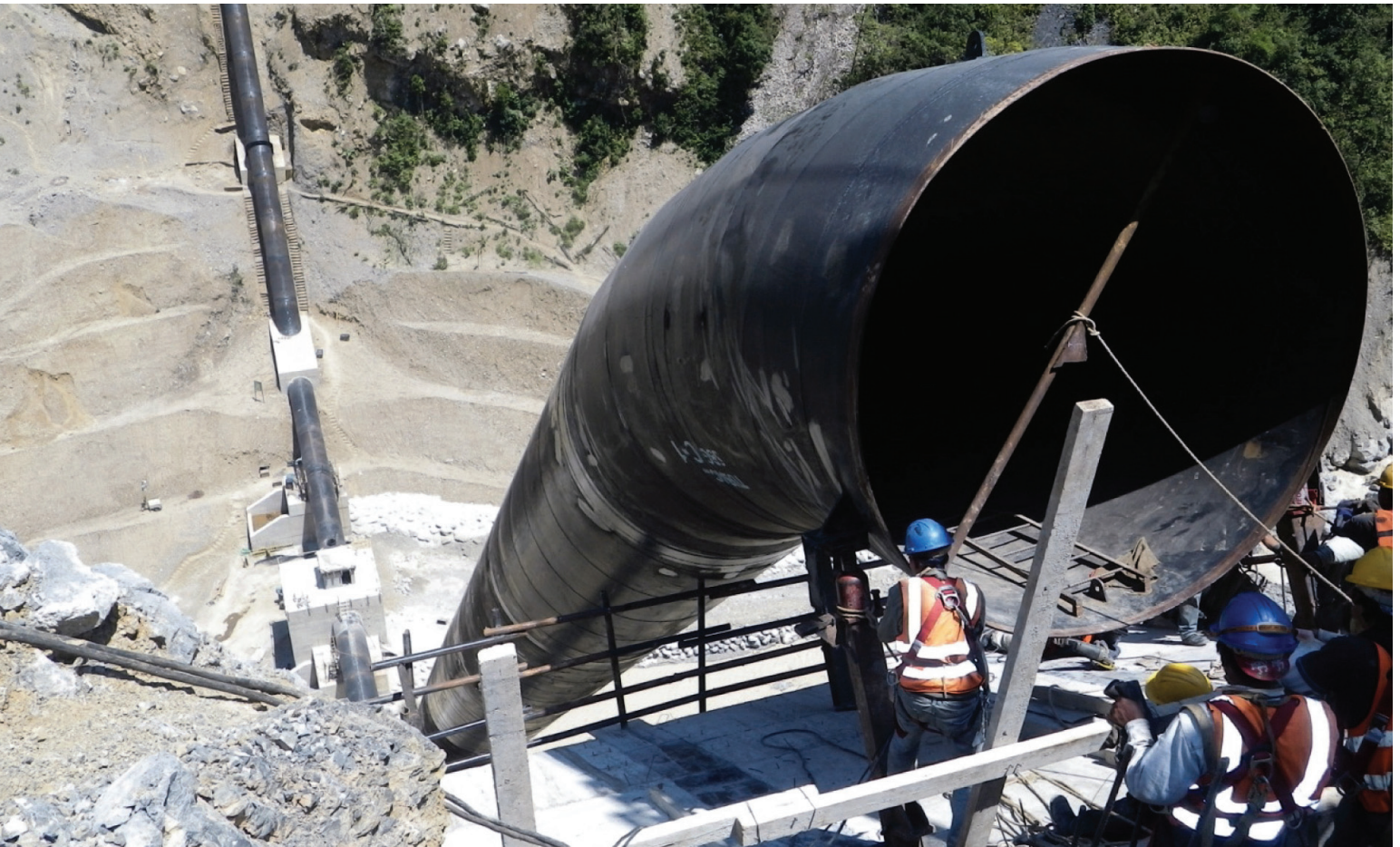
Regadio siphon - under construction
