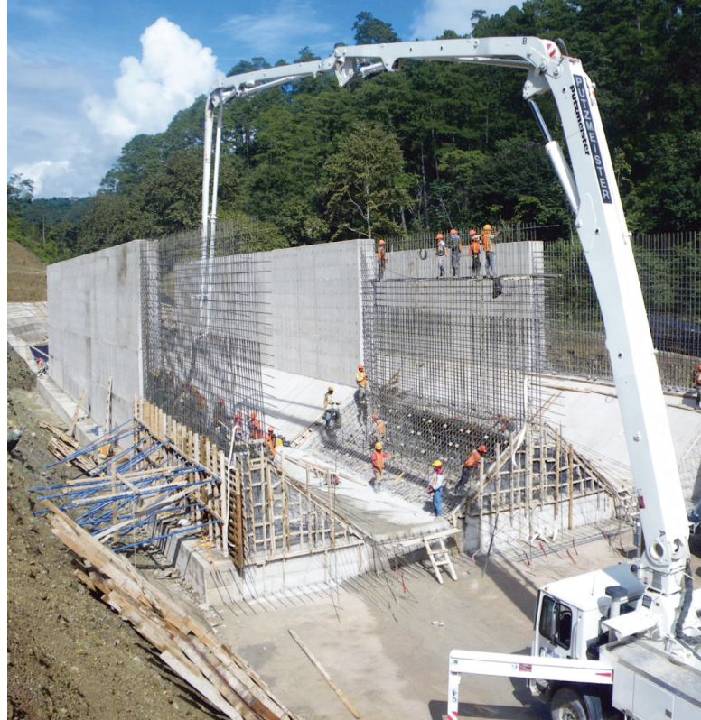
Cotzal desander - under construction
