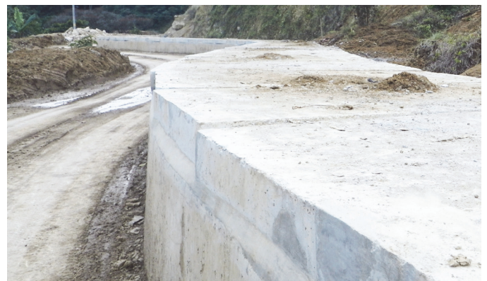
Landslide canal protection
