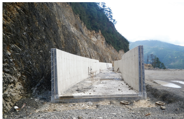
Construction of a rectangular canal
