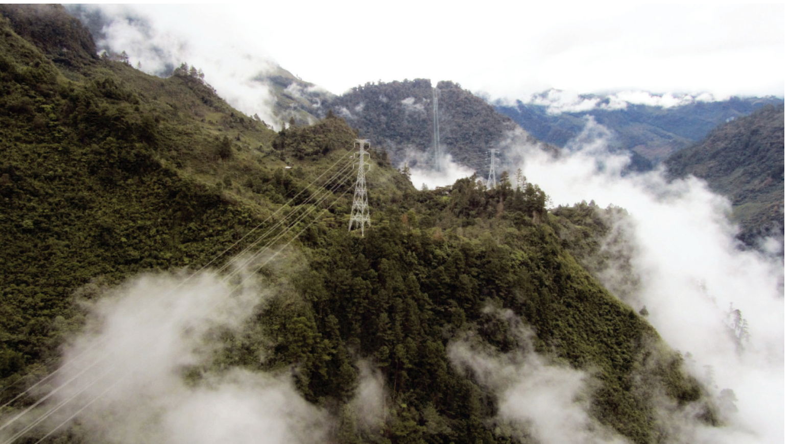
230 kV Transmission line transversing the Guatemalan Highlands
