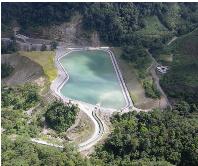
Off-river reservoir - 305,000 m 3 capacity
