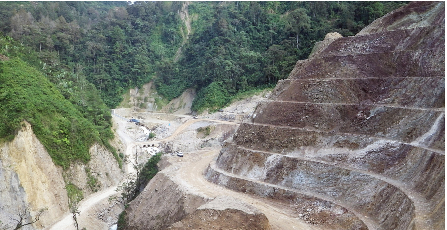
Landslide resistant slope excavation
