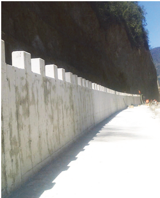
Overflow spillway protection
