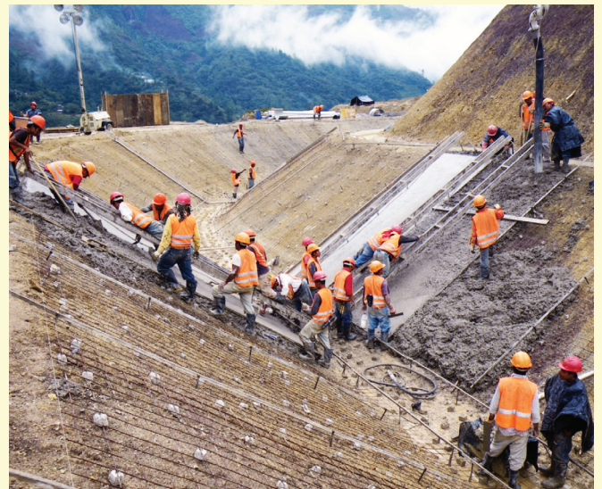
Typical construction activity along canal route
