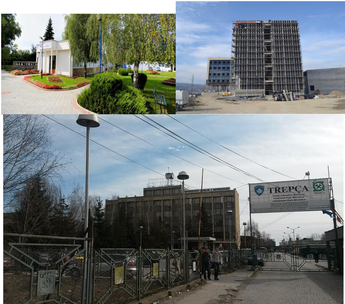
Figs. 67, 68, 69. University of Mitrovica ‘Isa Boletini’ (UMIB) [ Universiteti i Mitrovicës ‘Isa Boletini’ ], vice chancellor’s office building, the construction site of the dormitories, current teaching building of the university.
