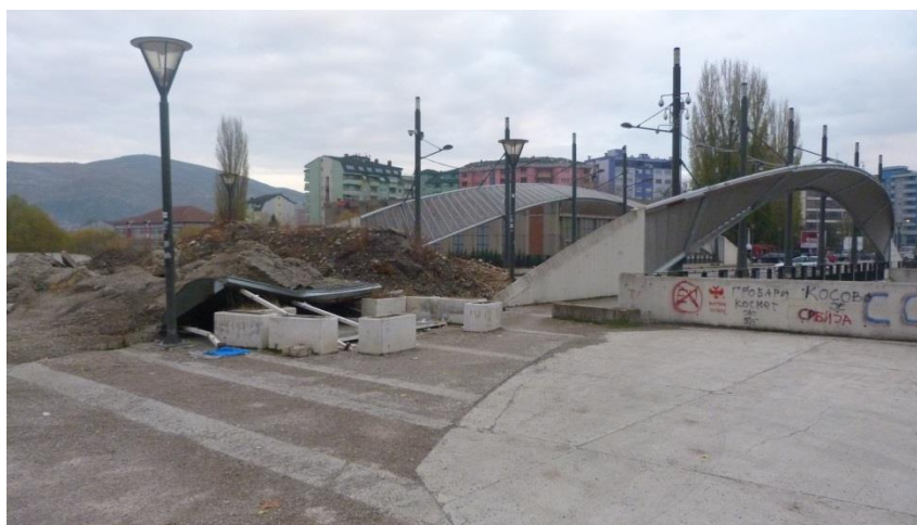
Fig. 13. The main bridge. North Mitrovica. Fieldwork November 2012
