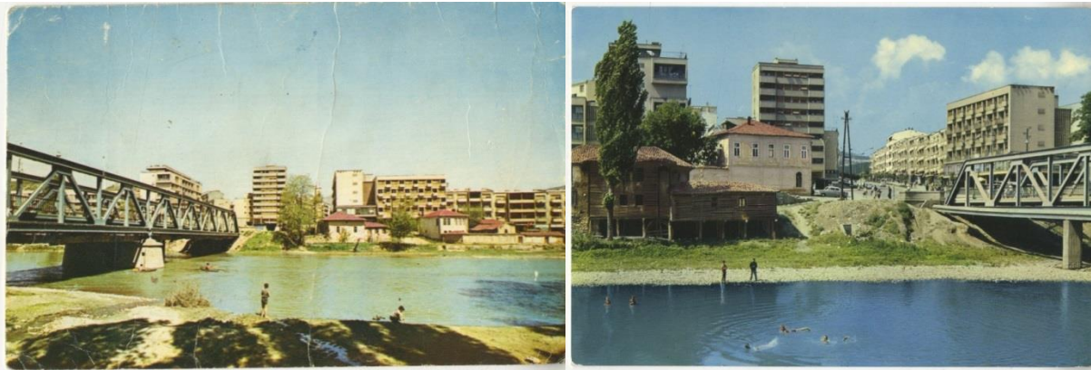
Figs. 11, 12. The main bridge in Mitrovica. National Library in Belgrade, Rg 174-007, Rg 174-019
