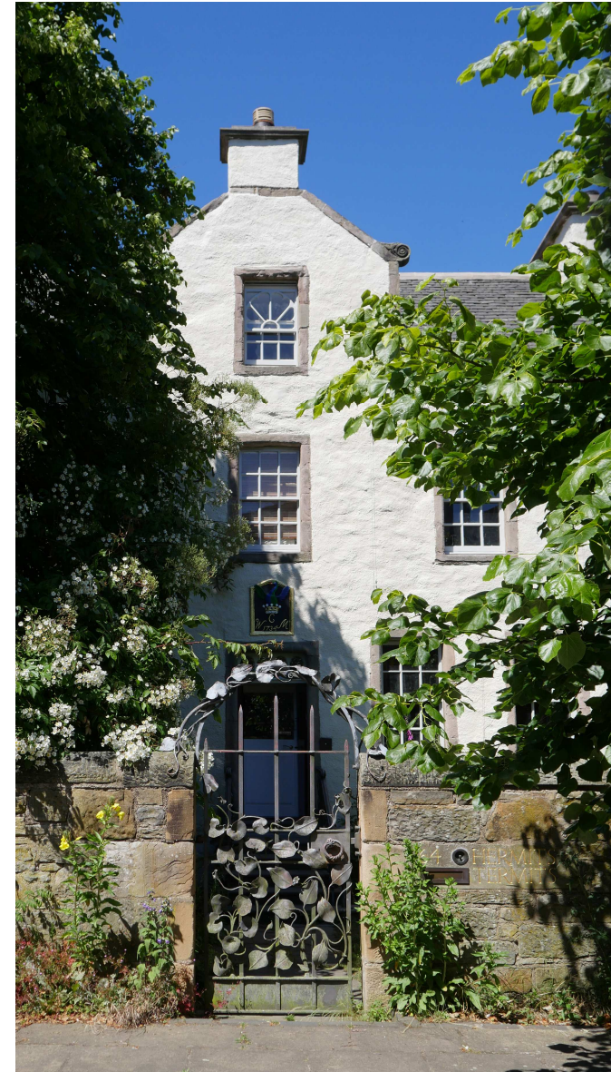
Lined render removed, replaced with lime harling based on historical evidence.
