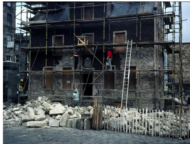
Lined render removed, replaced with lime harling based on historical evidence.
