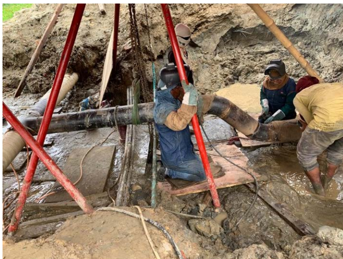
Pipeline construction work
