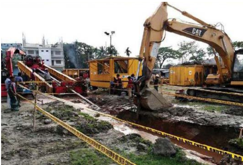
Brahmaputra River Crossing works through HDD method
