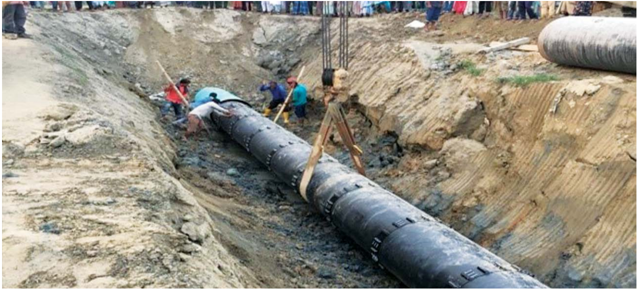
Road crossing activities under Chattogram-Feni-Bakhrabad Project of GTCL
