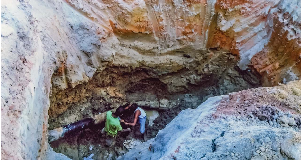
Gas pipeline leakage repairing activities of TGTDC
