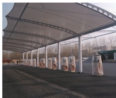
小营充电站 Xiao Ying Charging Station
