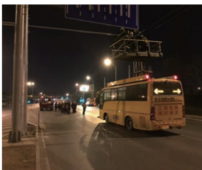
正在架设中的双源无轨电车线网 Dual-powered trolleybus power supply cable under construction
