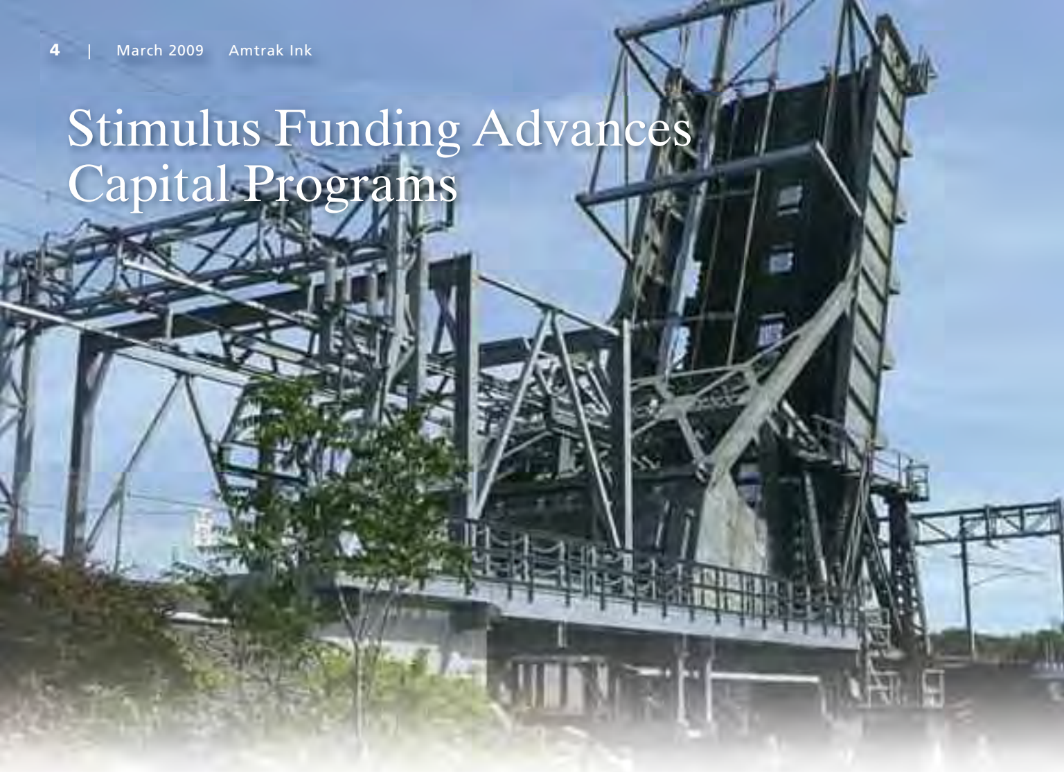
The Niantic River Bridge is one of several capital programs likely to benefit from stimulus funding.
