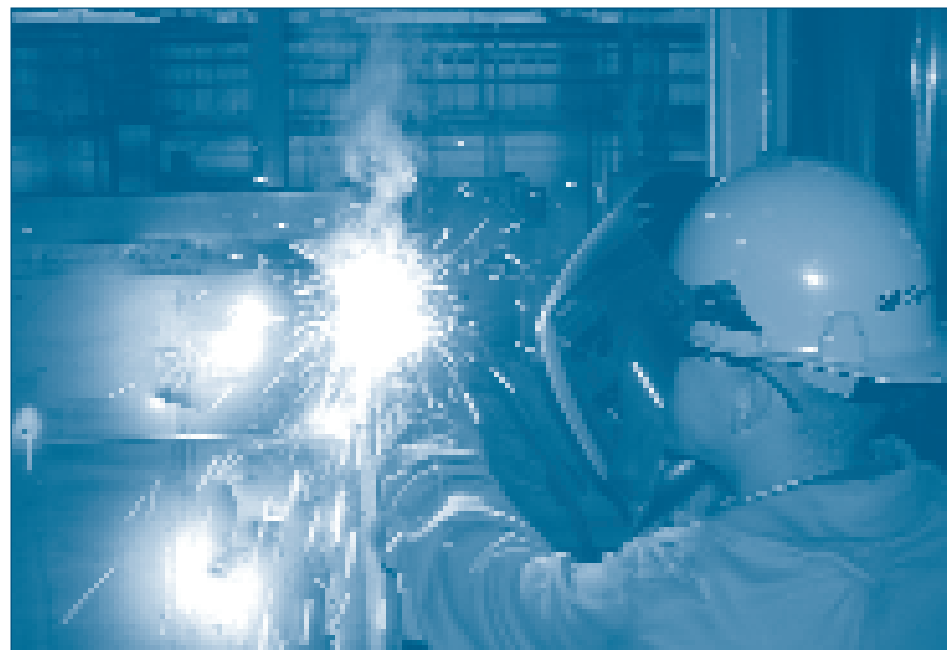
Frank Armstrong, car repairman at the Bear Car Shop, welds a steel reinforcement to a seat frame. Through new efficiencies and better tools, the Seat Shop Team produces seats for the entire system.
