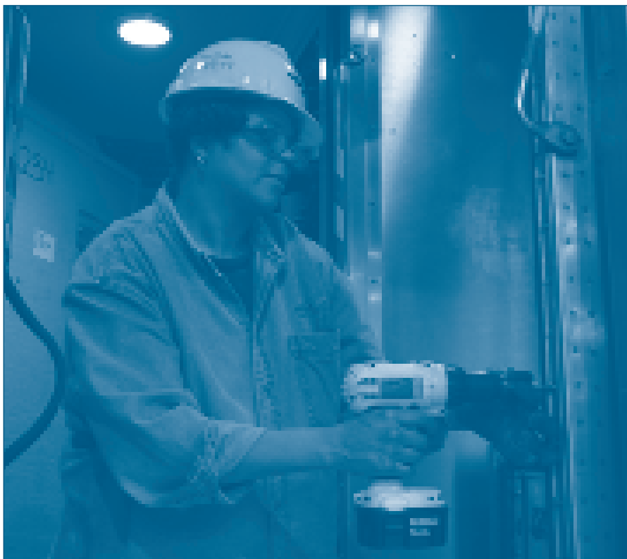
Car Repairman Vanessa Thomas replaces the weather stripping on the collision post door on Amfleet I Coach Car 44943.
