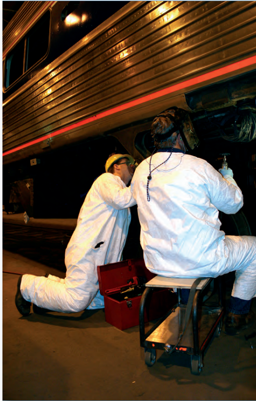
Bear maintenance facility employees work on an Amfleet car. The work being done by employees at the facility will result in returning 60 Amfleet cars to revenue service.
