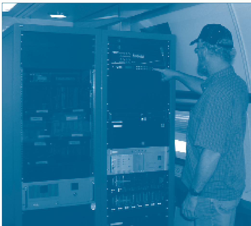
Inside the Track Geometry Car, Engineer of Rail Stress Management Marty Perkins sets parameters on the computer rack to display track measurement data for Maintenance-of-Way personnel. The computer rack contains the processing system that records track geometry measurements collected as the car operates on the system.
