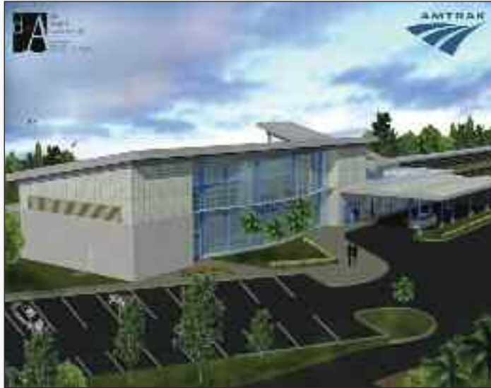
With a sloped shed roof line, the new Sanford station will resemble the Auto Train station in Lorton, Va., and include energy-saving lighting and HVAC systems, insulated glazing systems and other “green” features. Construction begins later this summer.
