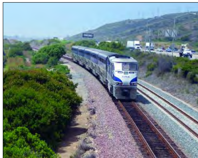
Photo: John Eschenbach A Pacific Surfliner train travels along the original main track, which runs adjacent to new continuous welded rail and concrete ties installed during the O'Neil-to-Flores project.
