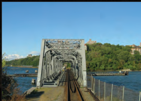
Train 235 approaches the Spuyten Duyvil Bridge in the Empire Division on Sept. 29, 2005.
