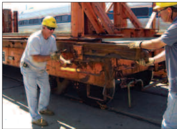
Photo: Stephen Reader At Bear Maintenance Facility, Repairmen/Inspectors Bobby Dean and Mark Flowers inspect the slide rail on Tie Car 15588.
