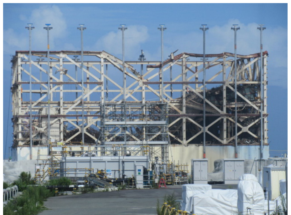
Photo: Tokyo Electric Power Company
