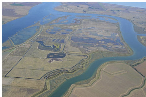
Aerial view of Wallasea Island 2019 looking east © RSPB
