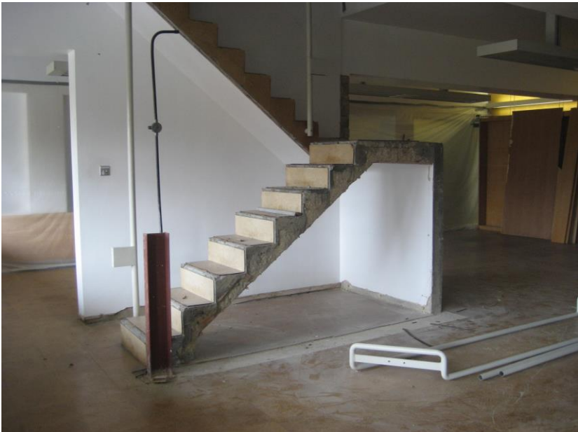
Building refurbishment in the Graduate Reading Room, July 2011. (BLL staff)
