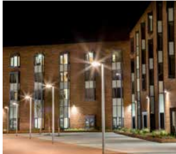
Grosvenor House student accommodation.
