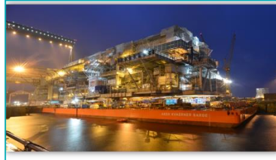
Load out and jacking November 2017
