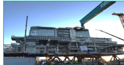
Accommodation modules installed January 2018
