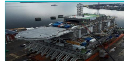
Heli deck & heli-hangar March 2018
