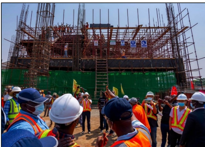
Construction of Oyingbo Station
