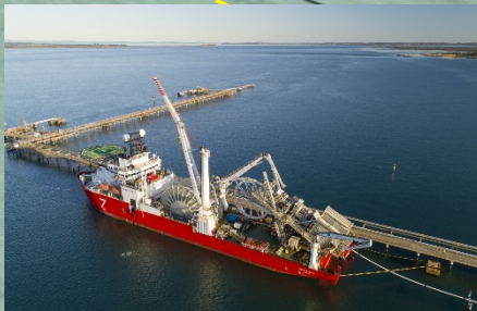
Subsea pipeline loading, Crib Pt Expected to complete Oct 18
