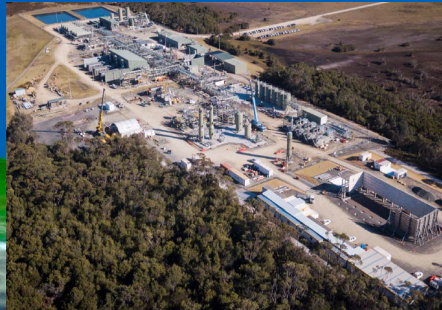
Orbest Gas Plant: Inlet gas area
