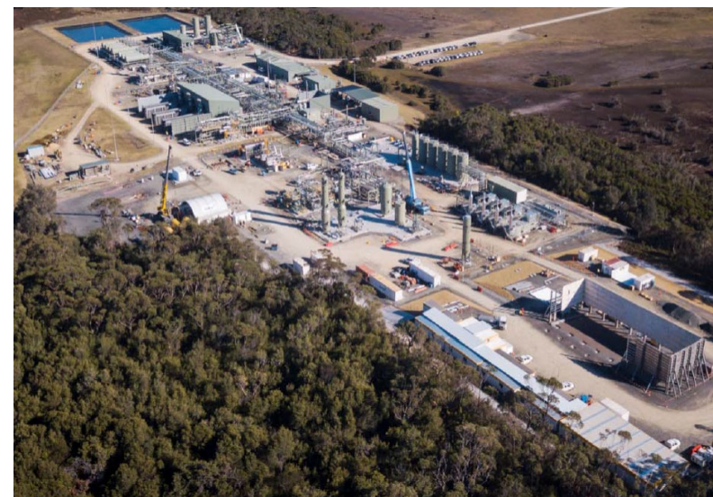
Orbest Gas Plant site works (APA Group)
