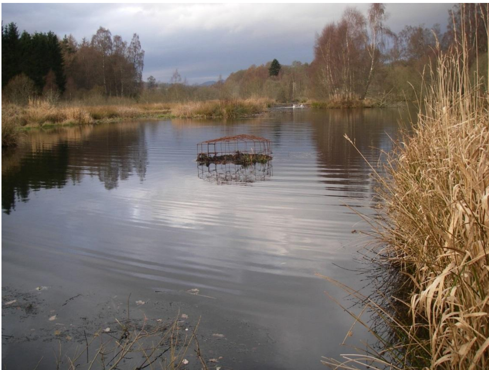
Figure 41. Cage protecting inflow end of pipe, set back from dam
