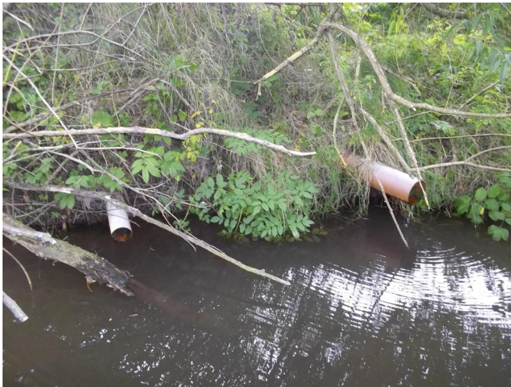
Figure 28. Field drainage pipes
