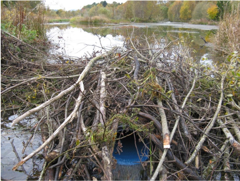
Figure 40. Dam constructed over pipe
