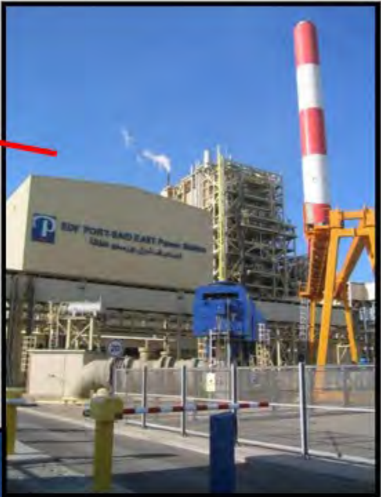
Port Said East Power
