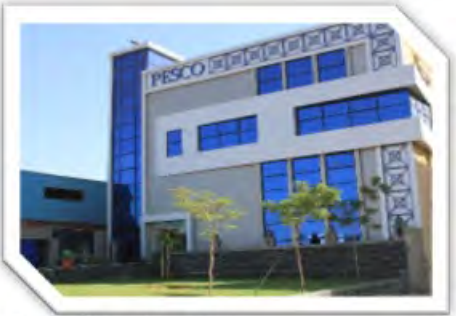
Egypt Office - New Cairo
