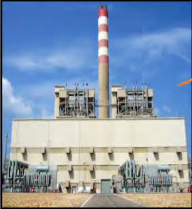
Sidi Krir Power Plant
