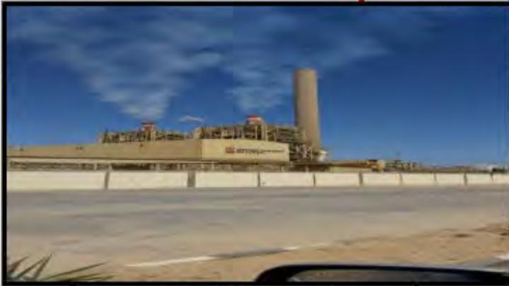
Suez Gulf Power Plant
