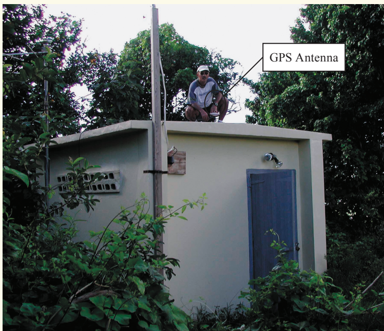
Base station (Bayfords Farm) for the ground deformation network
