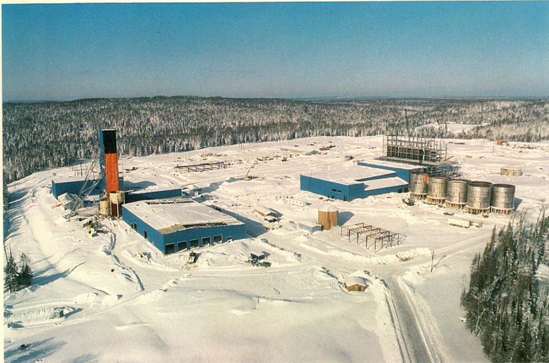
Aerial view of recent progress at Noranda's Hemlo site in January 1984.
