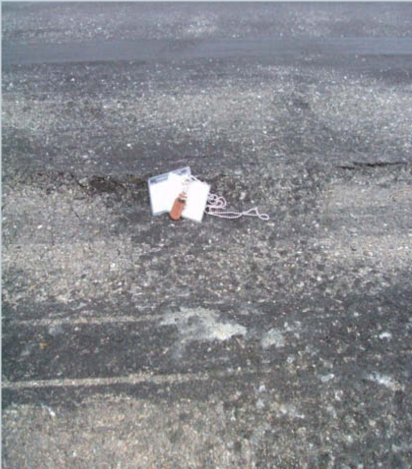
Runway condition before overlay
