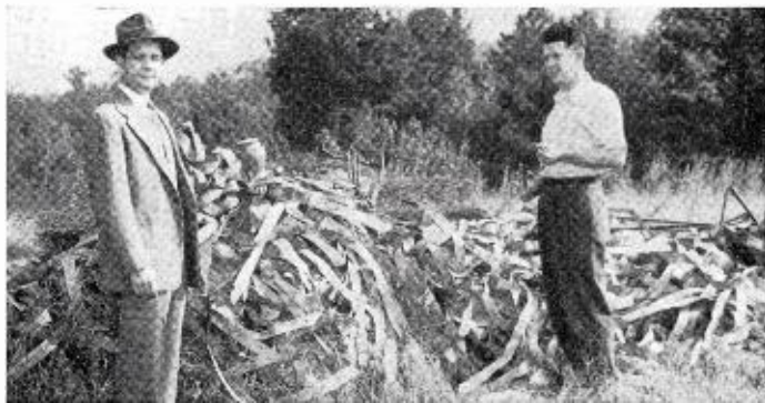
OUT OF THE TURF came 50,000 feet of pure copper ribbon and more than 300 pounds of 99% aluminum, recovered from the old 5,000-watt towers of WPTF, Raleigh. Richard Mason WPTF manager (left), and Henry Hulick, chief engineer, are looking over the ribbon pile just before it was carted away by Raleigh scrap campaign workers.
