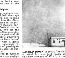
LASHED DOWN to resist Canadian wind, hell and high water is this new antenna of GJKL, Kirkland Lake, Ont. It is a Lingo guyed tubular steel vertical radiator 294 feet high. It is guyed at five elevations in four directions, spaced 90 degrees. The guys at the two upper elevations are high strength Copperweld steel strand % inch diameter. Those at the three lower elevations are extra high strength Copperweld strand ½ inch diameter.
