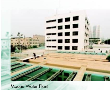
Macau Water Plant
