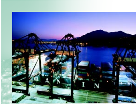
Container Terminal 3, Kwai Chung
