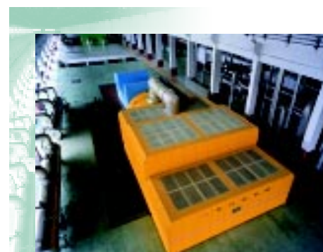
Zhujiang Power Station
