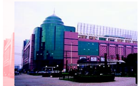
Tianjin New World Anderson Centre
