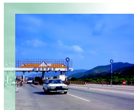
Shenzhen – Huizhou Roadway
