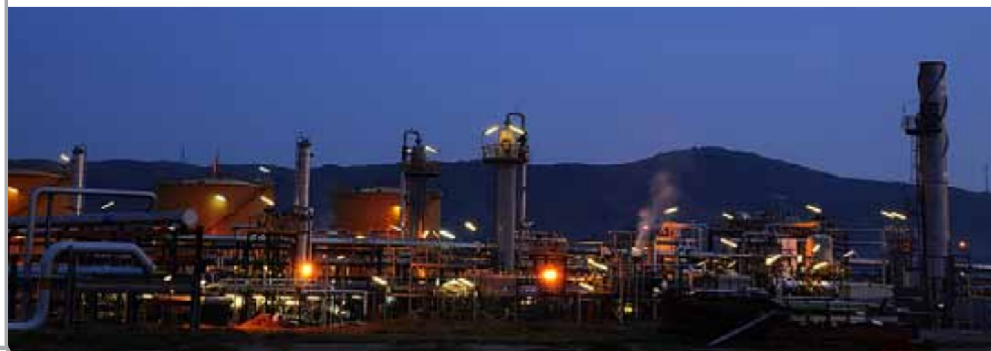
Manzalai Central Processing Facility, Pakistan
