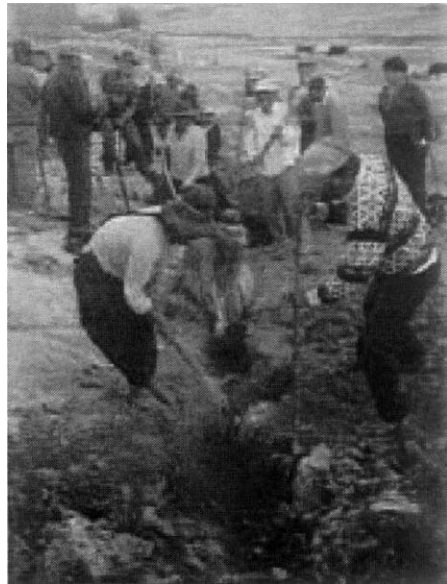
Community members dig water line in Huancarani, Peru.
