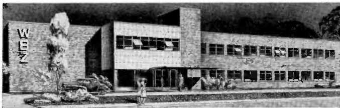
Television and FM activities of the Westinghouse Boston stations, WBZ and WBZA, will be housed in this $1,000,000 building of functional design now under construction adjacent to Harvard stadium.
