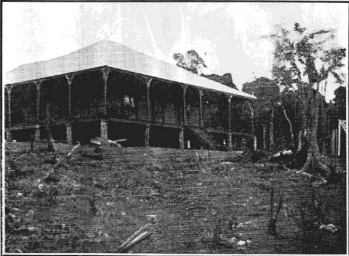
Superintendent's quarters at the Hull R. Aboriginal Settlement
