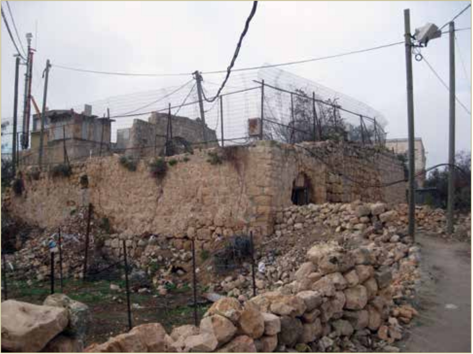
Dir el-Arba'in compound – Army lookout post
