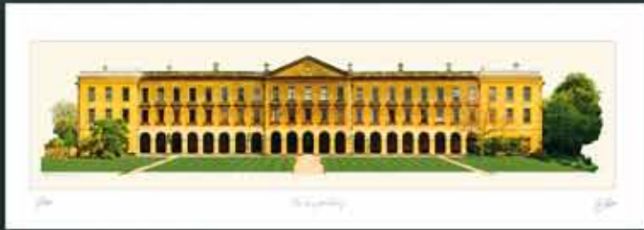
Magdalen The New Building
