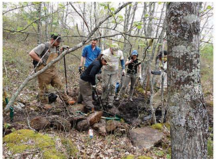
Treading Lightly: Trail volunteers learn how to build stone tread over wet spots.
