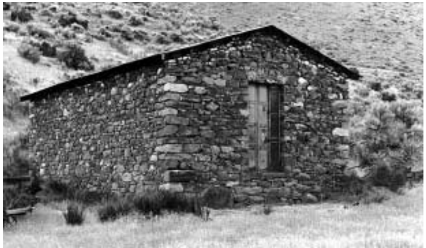
Stone building at Black Rock Crossing, Bruneau Canyon.
