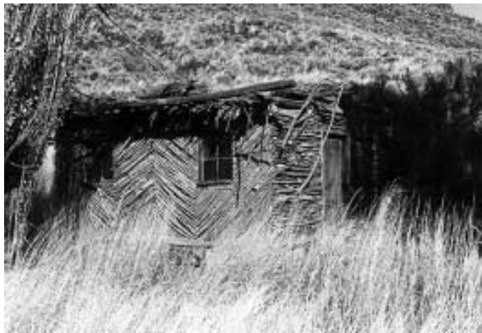
Primitive cabin at Roberson Place along Sheep Creek.
