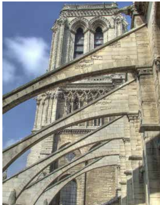
Figure 4.4 Ice shelves act like the flying buttresses used in some Gothic churches. The photo shows the buttresses on the Notre Dame Cathedral in Paris.
