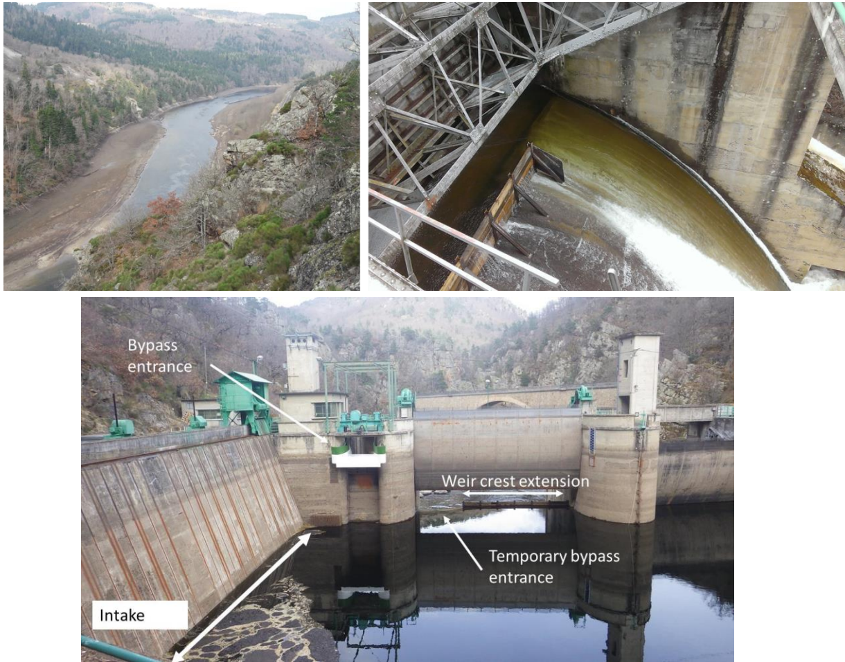
Figure 2.1.3: Top-left, picture of upstream limit of the temporary Poutès reservoir. Top-right, top view of temporary bypass. Bottom, upstream view of intake, usual (non-functional) and temporary bypass entrances.
