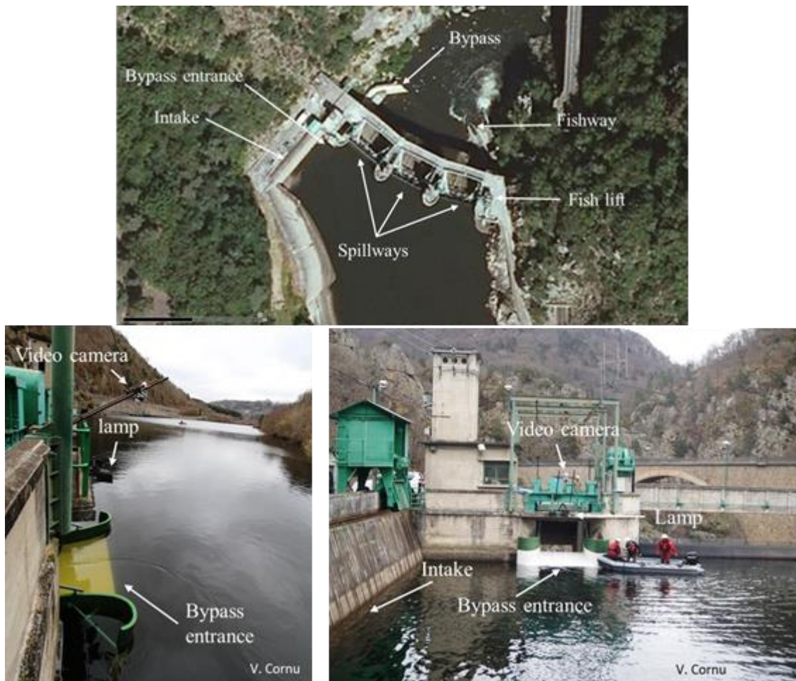
Figure 2.1.2: Aerial view of the Poutès dam (top), side view of the bypass entrance (bottom left) and front view of the intake and bypass entrance (bottom right) (Tétard et al. 2019).
