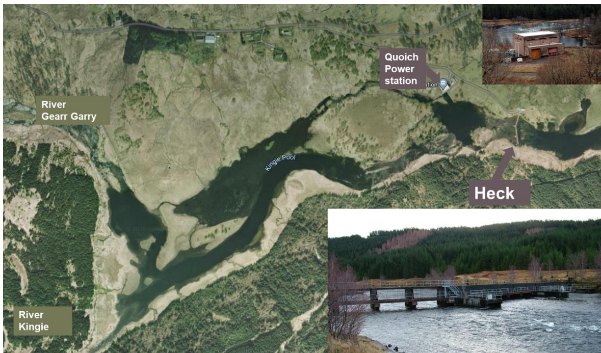
Figure 2.2.14. Fish barrier (heck) downstream of confluence between the Rivers Garr Garry and Kingie, and Quoich power station (photos overlaid on Google satellite image).
