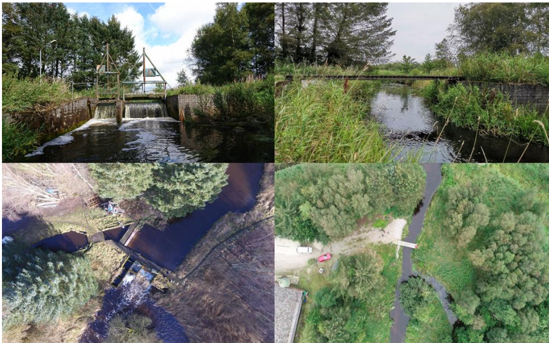
Figure 3.2.2. Trend Dambrug before (left) and after (right) removal.
