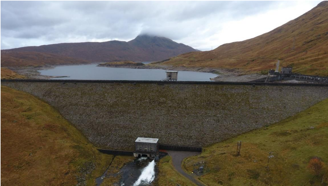
Figure 2.2.13. Quoich Dam – aerial drone photograph 2018 (taken by Shobhit Pipil, University of Durham).
