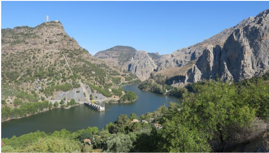
Figure 1.2.5: “La Encantada” (“El Chorro”) Dam.
