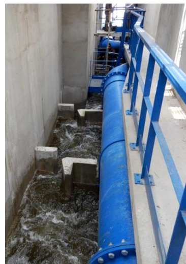
Figure 2.3.6. The fishway after modernization.
