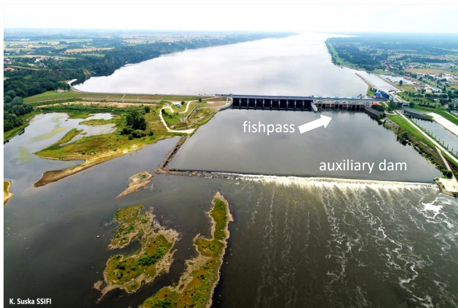
Figure 2.3.4. The Włocławek Dam on the River Vistula. The new fishpass marked with an arrow and the auxiliary dam.
