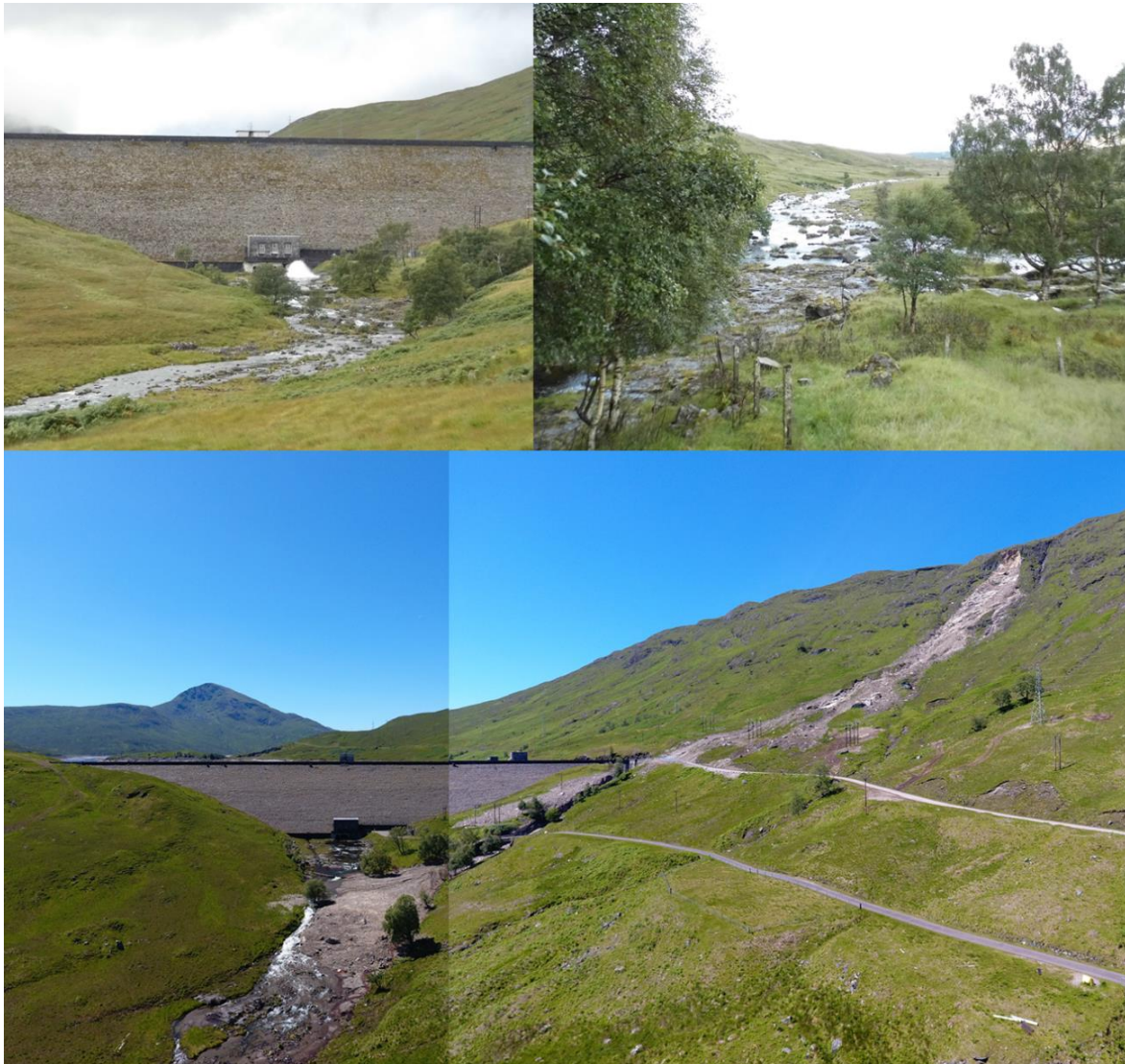
Figure 2.2.15. Landslide downstream of Quoich Dam (before and after). Top left: view of Quoich Dam in August 2017; top right: view from Quoich Dam spillway (same date); bottom: composite photo of Quoich Dam and landslide in August 2019.
