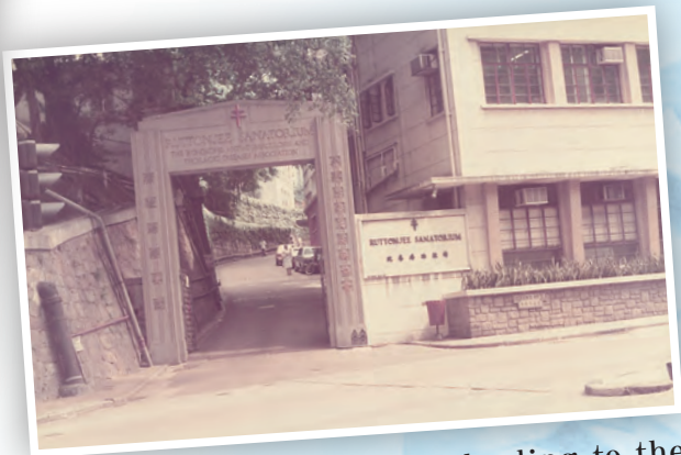
The former stone archway leading to the old Ruttonjee Sanatorium adjacent to the Association's Headquarters 早期香港防癆會進入律敦治療養院之拱門
