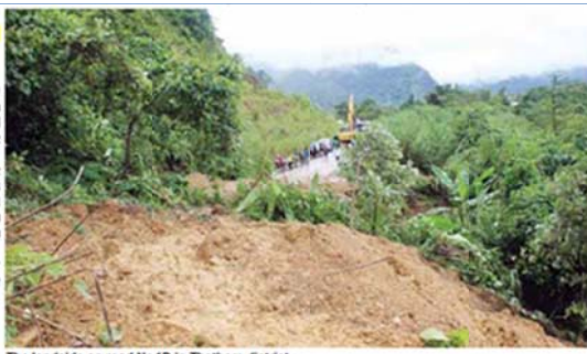
The landslide on road No.1D in Thathom district.
