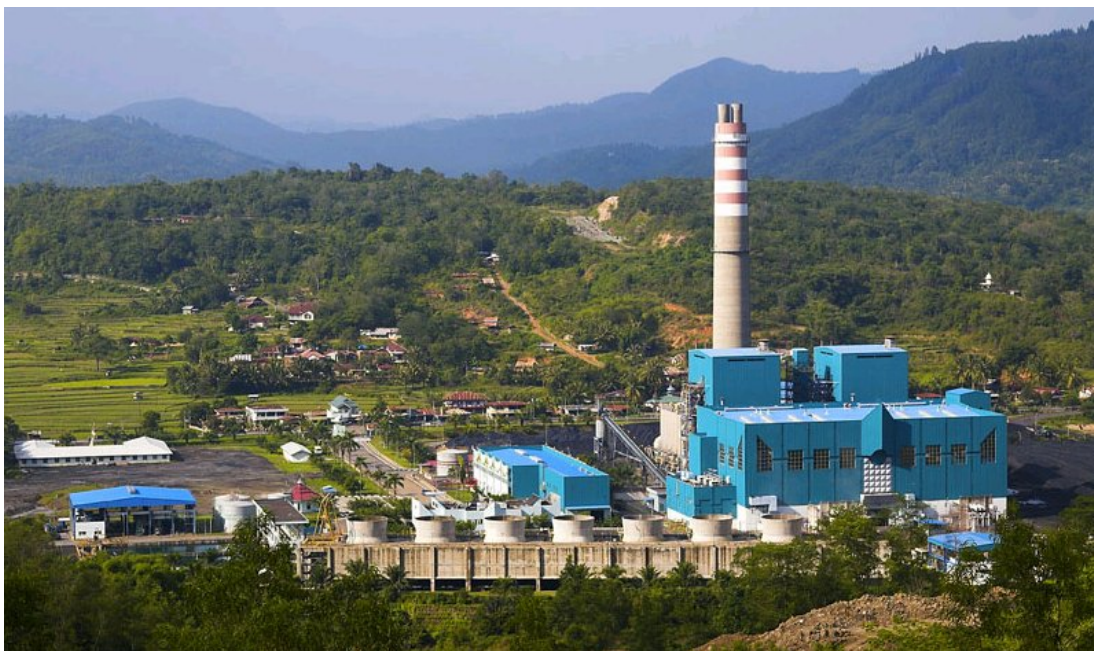
Figure 10.4. A view of Kandi Thermo-electric Power Plant
