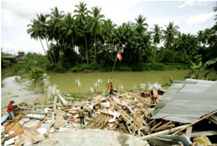
(b) Embankment failure along a river in Solok District Figure 8.7. Some views of embankment failures
