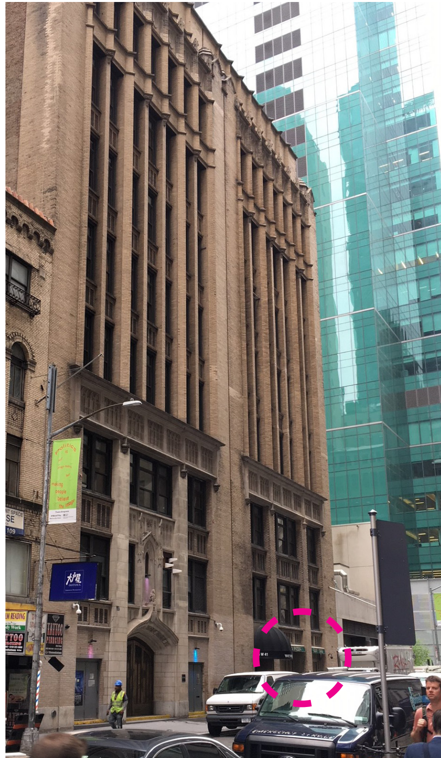
PHOTO TAKEN STANDING ACROSS THE STREET
