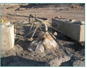
Paste Injection into Borehole
