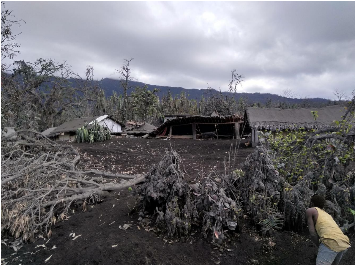
Figure 3 Heavy ashfall damage to crops and traditional buildings under ~150 mm ashfall, South Ambae. 8 August 2018. (Photo Credit: Carol Stewart)
