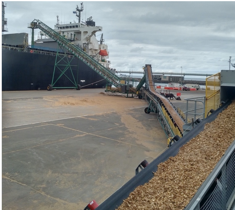
Figure 23 Case C - Wood Chip Vessel Loading Using Mobile Conveyor Systems
