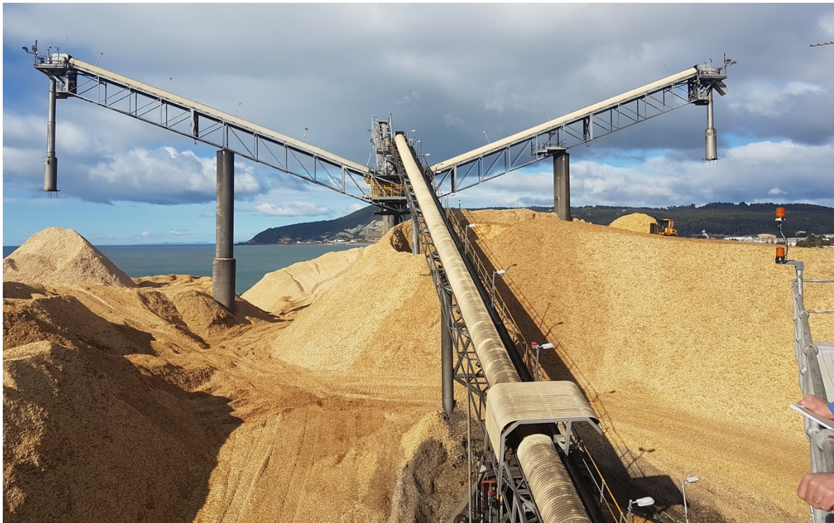
Figure 10 Case A - Wood Chip Storage at Marine Terminal
