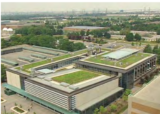
Examples of lot level stormwater management practices: bioretention swales, porous paving, green roofs, and rain gardens.
