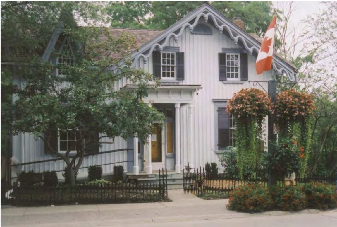
Kathleen McKay Art Gallery, Unionville (former Fred Varley home) – an example of adaptive re-use of a heritage building.
