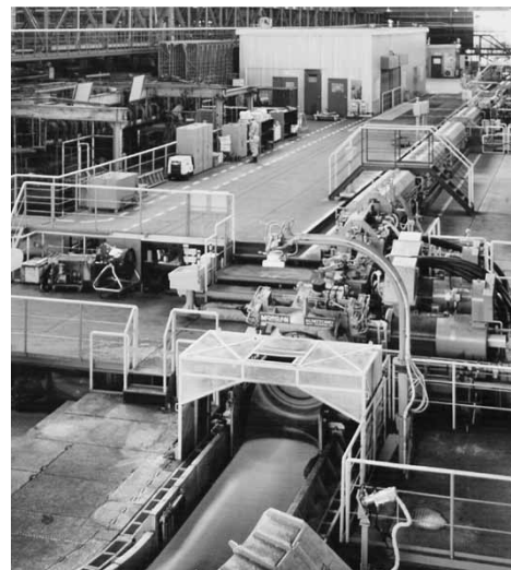
Fig. 5 Laying head of No. 7 wire rod and bar mill at Kobe Works
