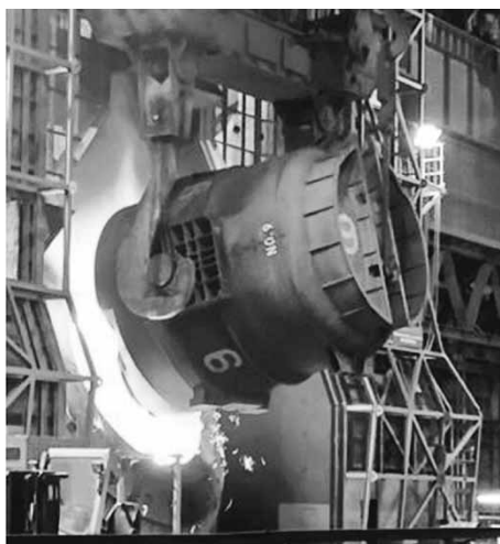
Fig. 1 New plant for molten iron treatment
