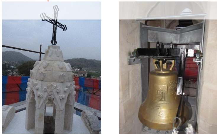
Figure 8: Restoration (left) and strengthening (right) of Saint John's bell tower in Psevdas (photos taken in December 2017)
