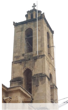
Figure 5: Bell tower of Saint John's Cathedral with timber ties, Nicosia
